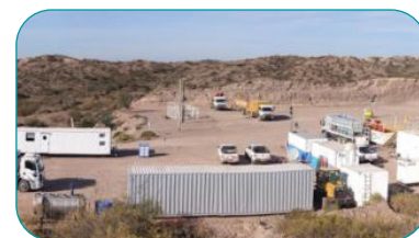
Fig 3: SWCTT injection and monitoring set-up
